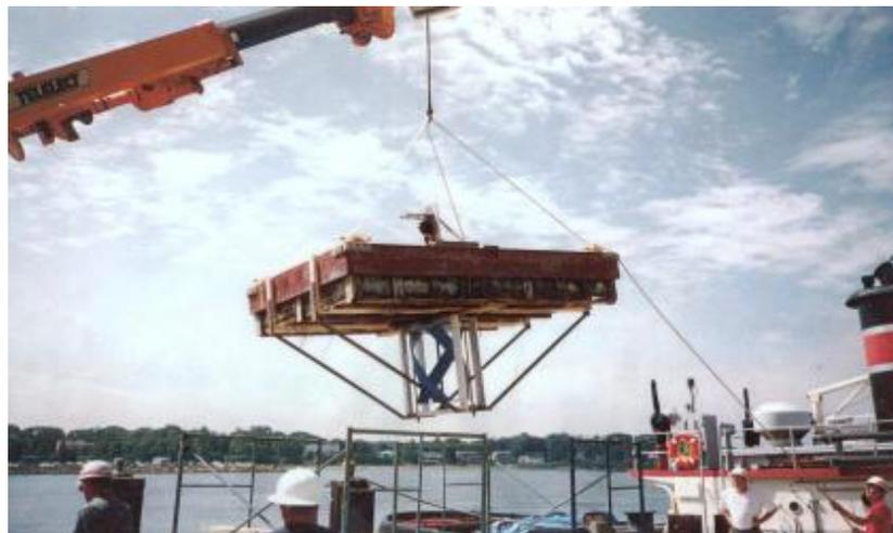
**Fig. 3** Installation of Triple-Helix Turbine in the Cape Cod Canal
